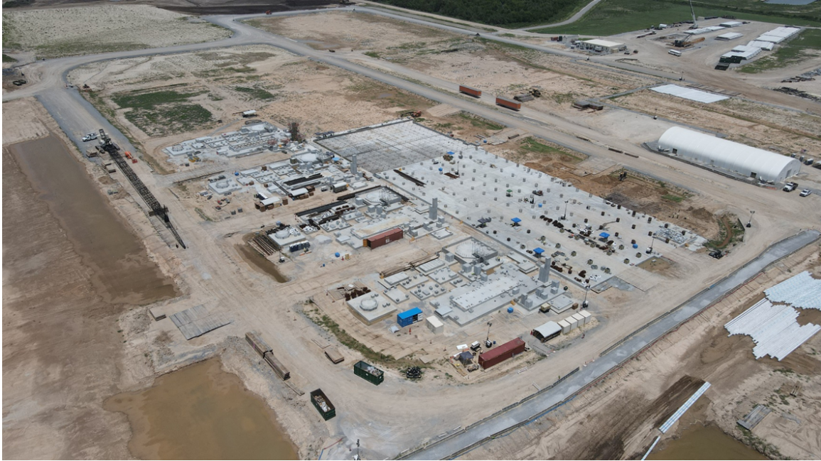
Driftwood LNG construction as of 13 July 2023
